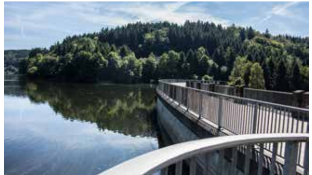
Raw water for drinking water supply.
