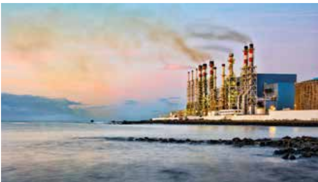
Raw water for seawater desalination.
