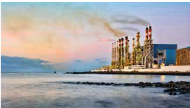
Raw water for seawater desalination.
