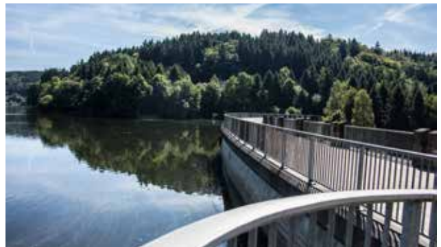
Raw water for drinking water supply.
