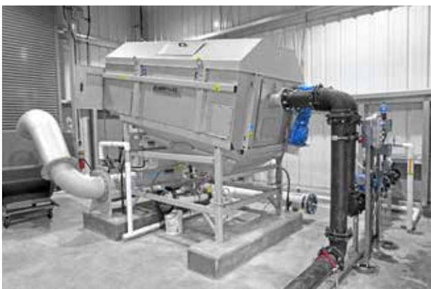
HUBER Sludge Acceptance Plant RotaShield® in use.
