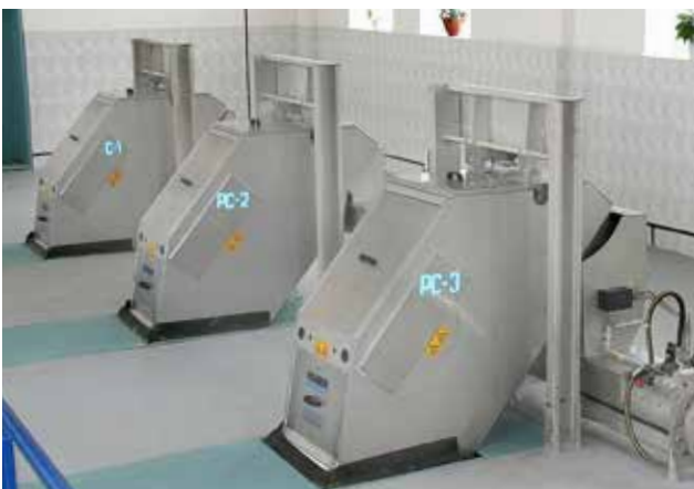
Use HUBER Fine Screen STEP SCREEN® SSF in Russia: pivotable in the channel without having to remove the downstream HUBER Wash Press WAP® and HUBER Trough Screw Conveyor.
