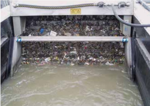
HUBER Fine Screen STEP SCREEN® SSF – L= 3500, W=1826, 6 mm slot width, installation angle 50°. High capacity as the flow passes the screen surface only once.
