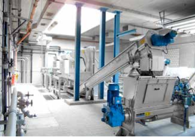
3 HUBER Step Screen STEP SCREEN® SSV units: L=4300, W=1176, 3 mm slot width. Optimally adjustable to suit specific constructional conditions (big discharge heights, deep channels) due to the steep installation angle of 70–80°.
