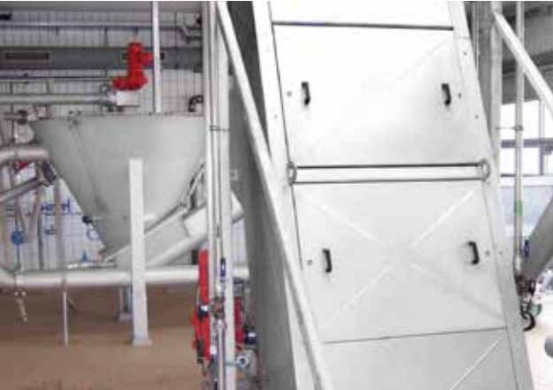
HUBER Fine Screen STEP SCREEN® SSV in channel, pivotable without having to remove the downstream HUBER Wash Press.
