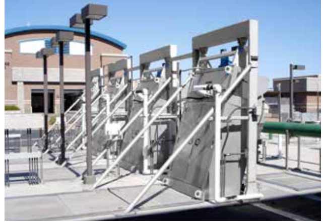
4 HUBER Fine Screen STEP SCREEN® SSV units: L=5300, W=1376, 6 mm slot width, installation angle 75°. Maximum operational stability due to the special bottom step design for increased operational reliability without impairment by grit, gravel, stones.
