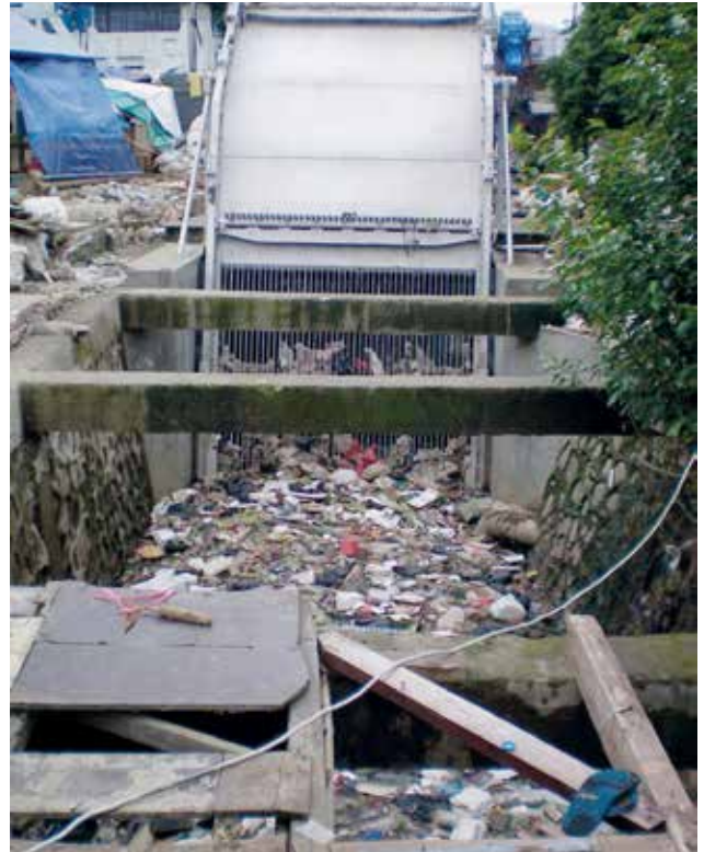
HUBER Coarse Screen TrashMax® in operation.
