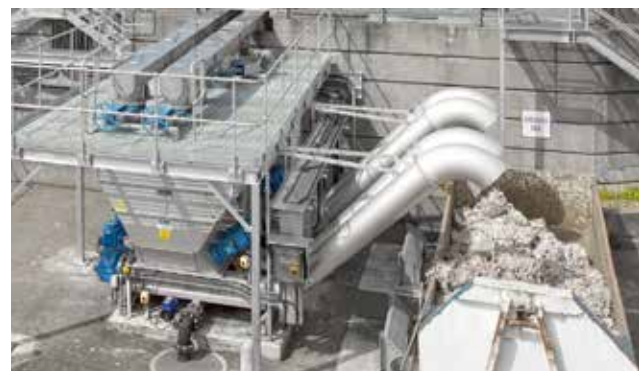
Washed and almost odourless screenings from a HUBER Screenings Wash Press WAP® SL.
