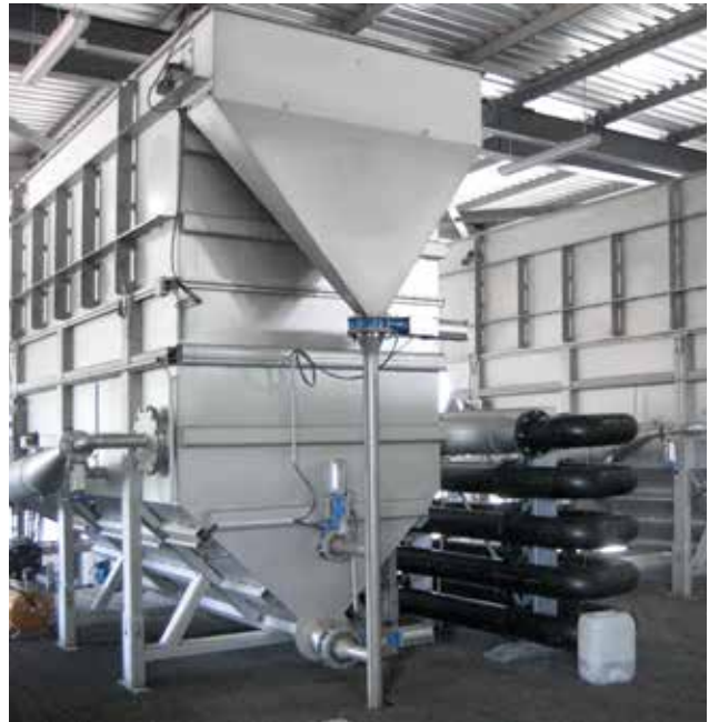
HUBER Dissolved Air Flotations Plants with chemical stage for activated sludge separation – the solution to relieve overloaded biological treatment plants.
