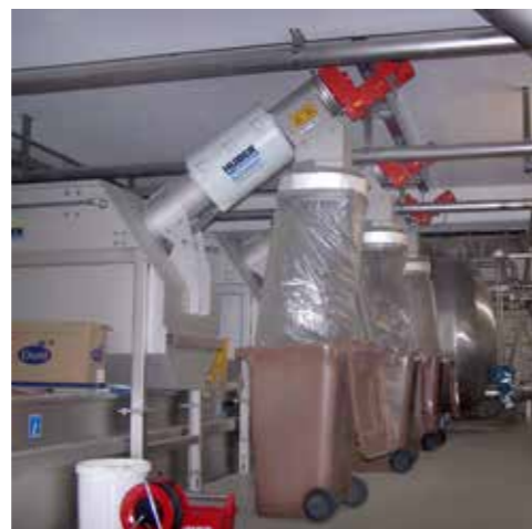
HUBER screens and fine screens as well as grit and heavy material separators for the best possible and project-specific mechanical treatment of wash water and production wastewater from breweries, the fruit juice industry as well as from the production of mineral water and other alcoholic and non-alcoholic beverages
