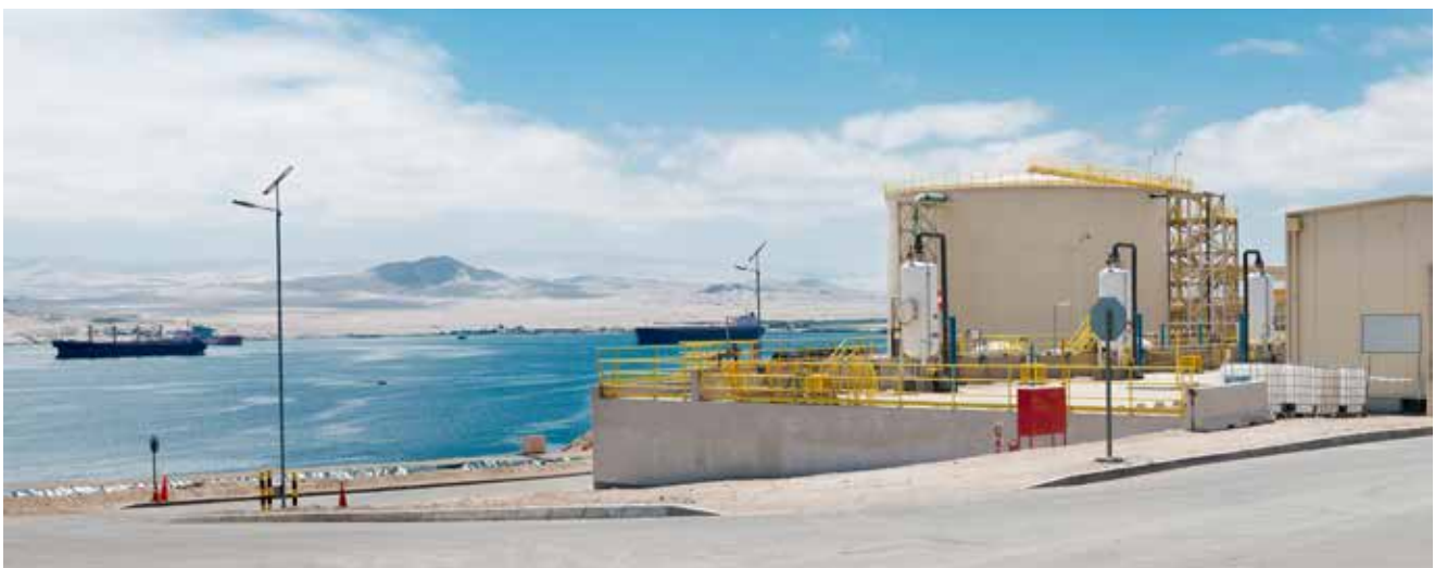
Desalination facility in the Punta Padrones Area, in Caldera City (Atacama)/Chile.
