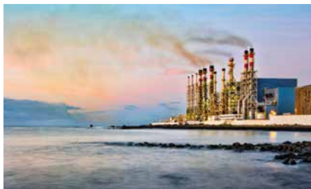
Desalination plant at Arrecife in Lanzarote.
