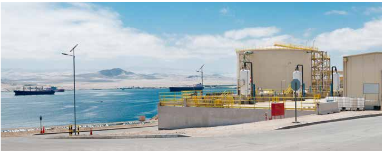
Entsalzungsanlage in der Punta Padrones Area, in Caldera City (Atacama)/Chile.
