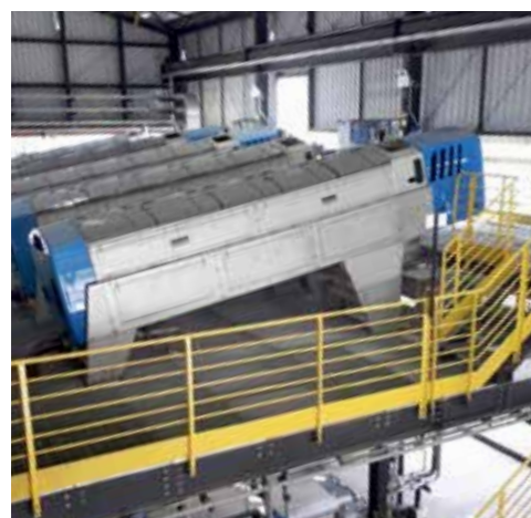
HUBER Screw Press units for sludge treatment – best dewatering performance and highest volume reduction for lower disposal costs.
