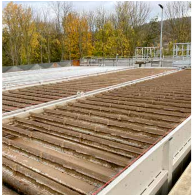
HUBER Dissolved Air Flotation Plants with chemical stage for secondary treatment – the solution to relieve overloaded biological treatment plants.
